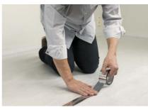
Protecting your floor against rising moisture is a must. We recommend you use Parky's tested waterproof tape to glue your underlay together. It's the only way to protect the backside of the floor.
